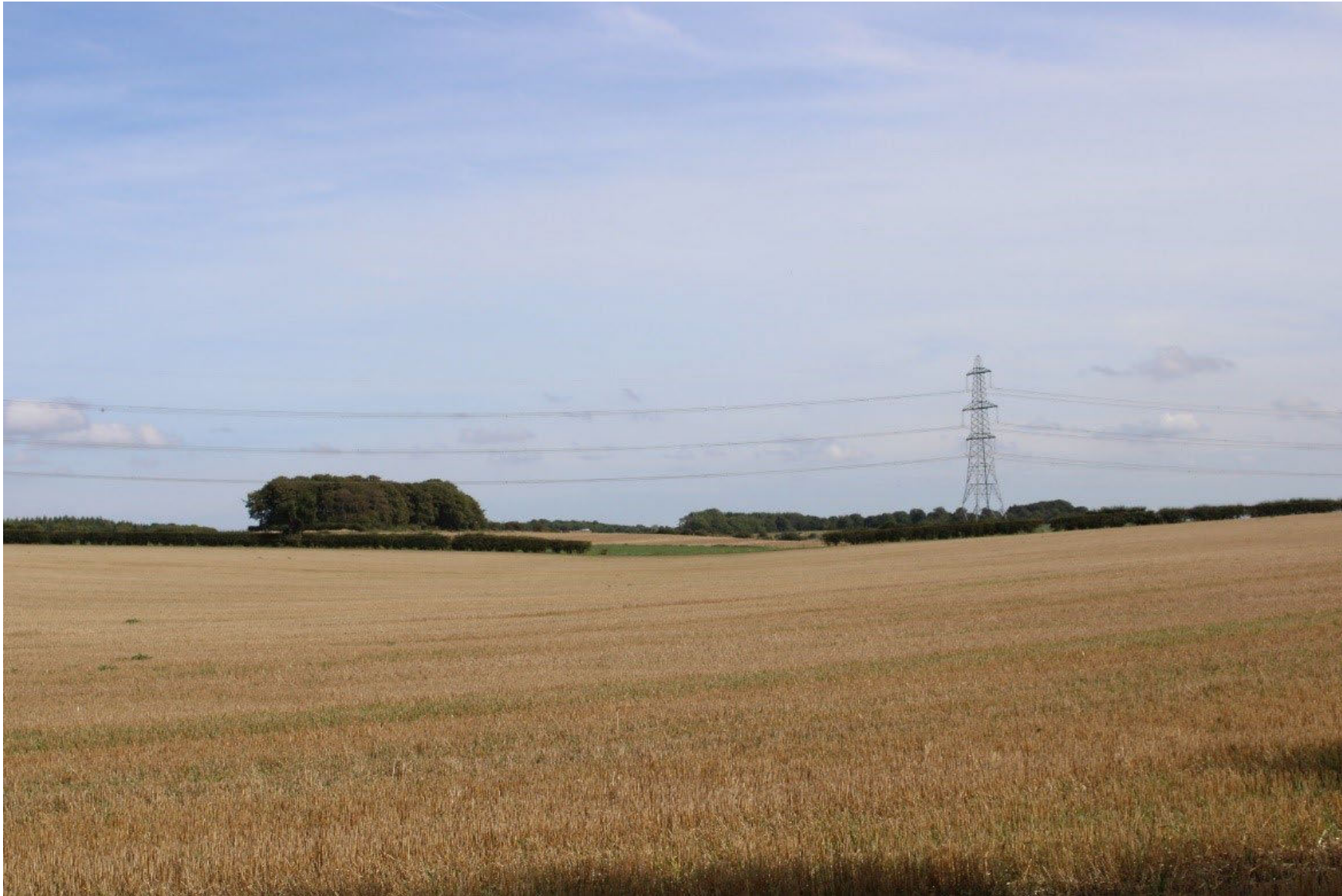
Illustration 3: General Shot of Springwell West looking east
